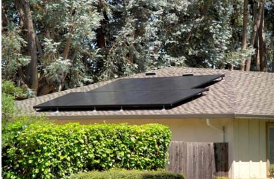
**Non compliant street-side roofs with exposed and metallic mounting hardware and lack of symmetry in application of equipment**
